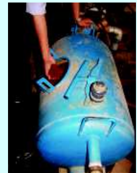
Cleaning of Sand filters
