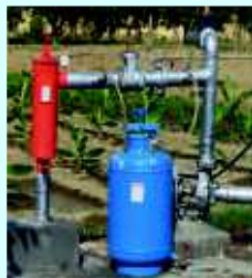
Installation of Drip Irrigation System
